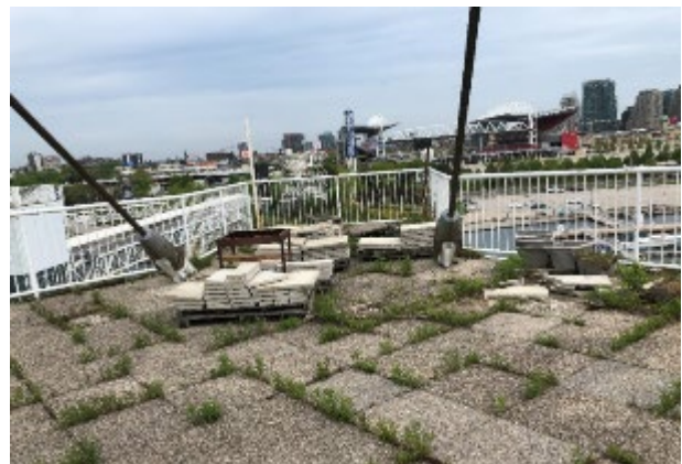
Figure 66: Photograph of the pavers on the Pod roofs. (Credit: ENTUITIVE 2020)
