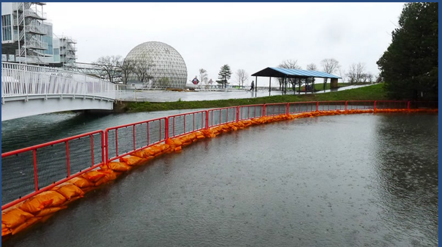
Recent flooding on site
