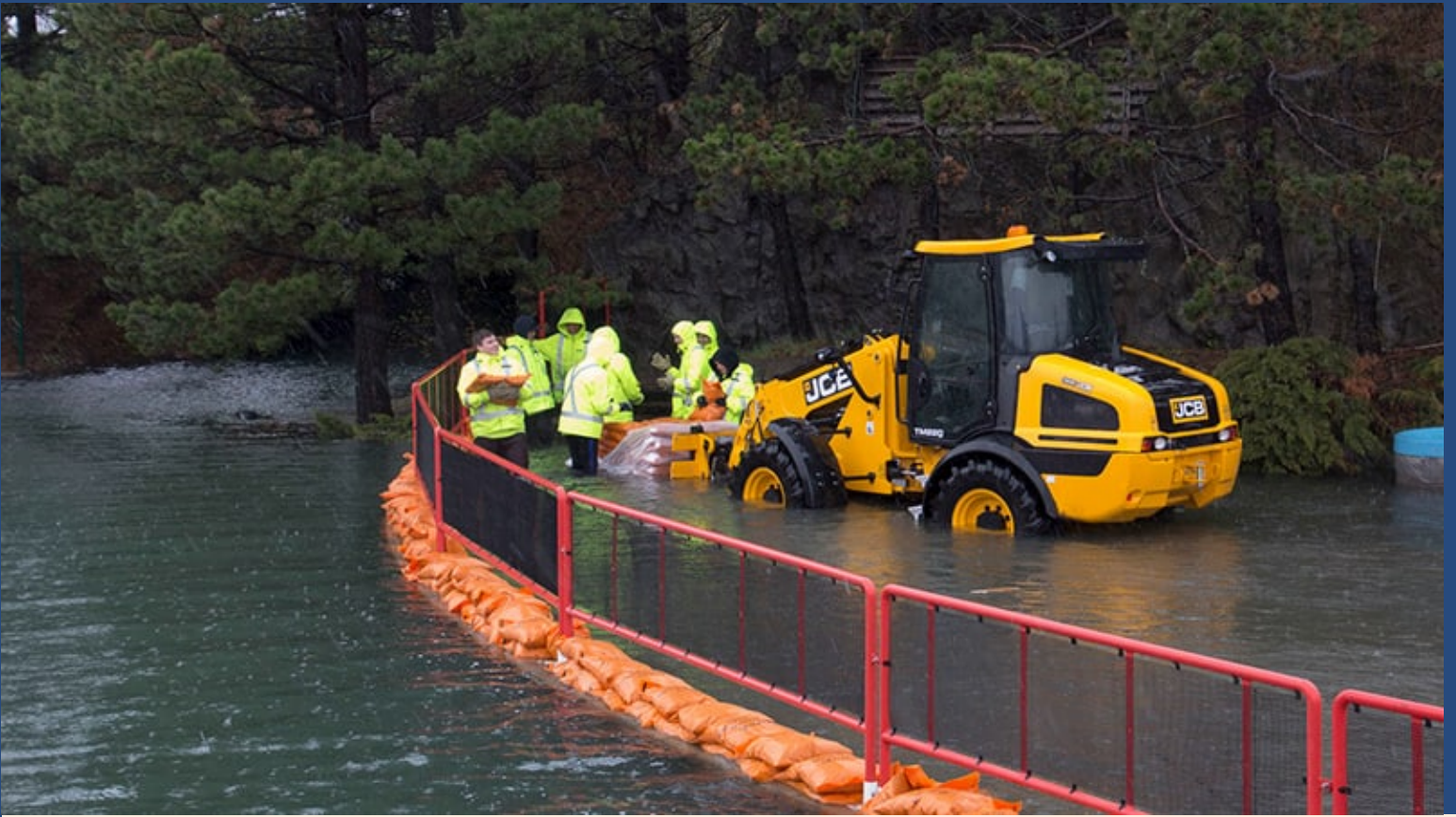
Recent flood repairs
