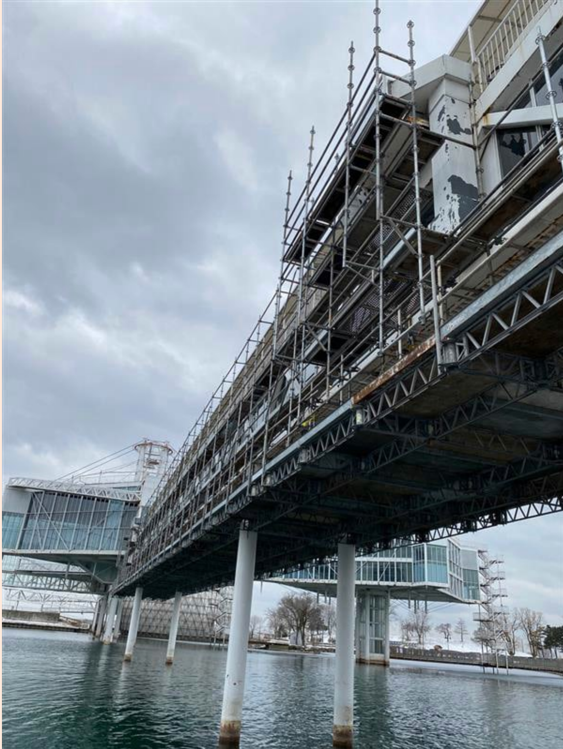
Scaffolding along a bridge to the pods.
