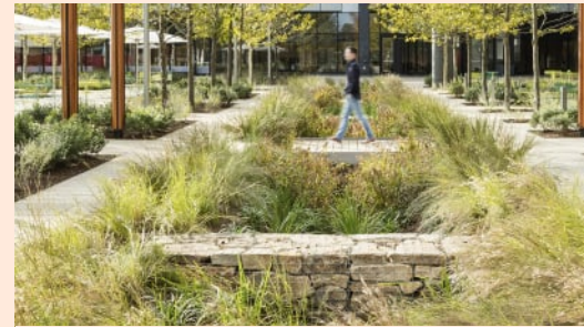
Naturalized stormwater management
