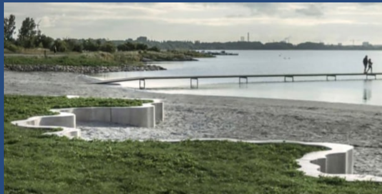
Reinstated Hough edge
