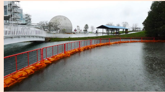
Flooding on site.
