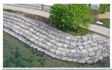
Figure 17: Example of terraced armour stone at Sunnyside (photo courtesy TRCA)
