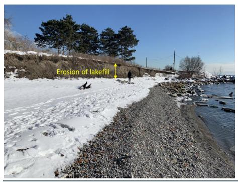
Figure 10: Significant erosion of lakefill at south shore (Baird 2021-01-30)
