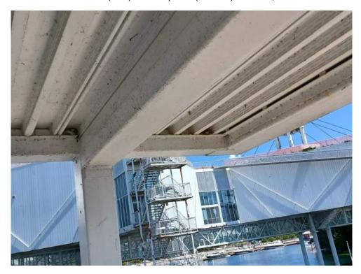
Figure 54: View of Cliff Swallow nests in grooves in underside of Secondary Tower Ramp Element 7 (SB7). June 23, 2022.
