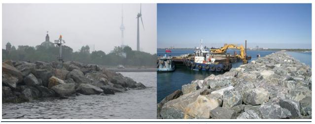
Figure 14: Armour protection at Western Beaches breakwater (Baird)
