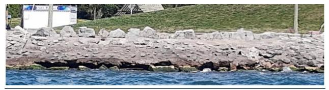
Figure 12: Deterioration of grouted stone revetment at east headland (from Jacobs, 2020)
