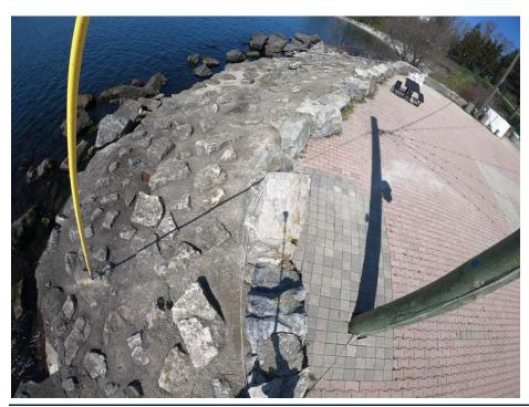
Figure 11: View of deteriorated grouted revetment at east headland (Baird 2022-04-29)
