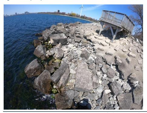
Figure 9: Damaged armour protection at west headland (Baird 2022-04-29)
