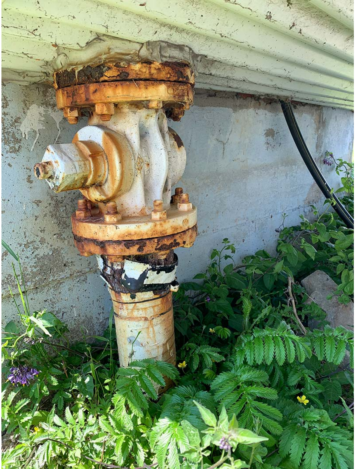
Corroded plug valve under Cinesphere bridge connecting to west marina. Photo from TYLin, June 2022.
