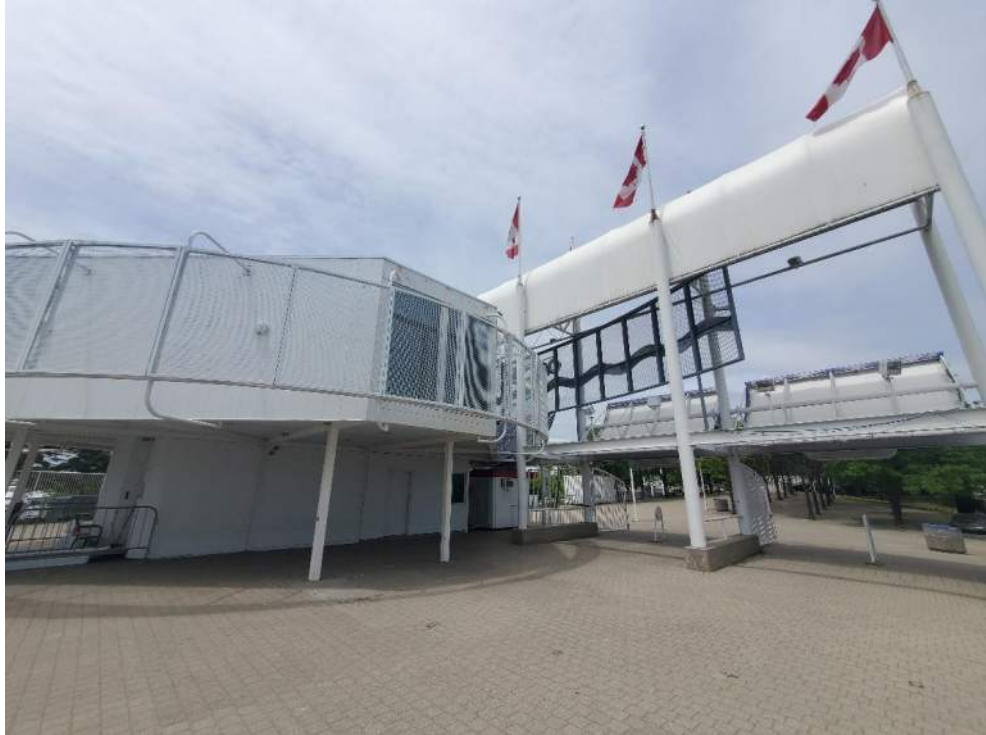
Figure 143: View, facing northwest, of the Central Entrance Offices (B92534) and the Central Entrance Structure (B92533). June 20, 2022.
