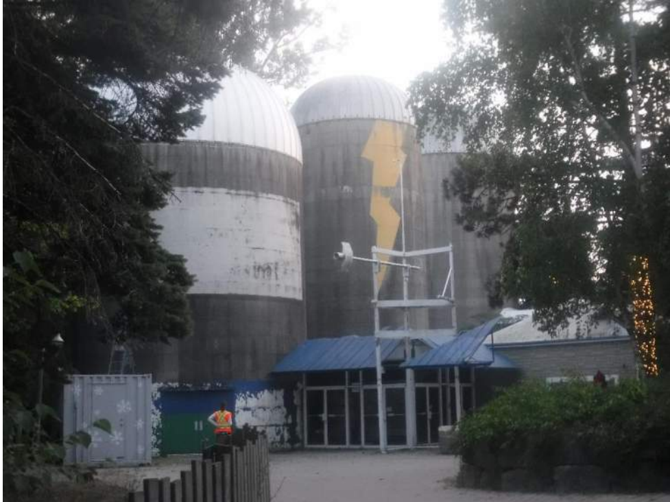
Figure 39: View, facing west, of the Silo Assembly Space (B92539), part of the Interconnected Silos Complex (B92538) and Bat Acoustic Monitoring Area #2. July 7, 2020.
