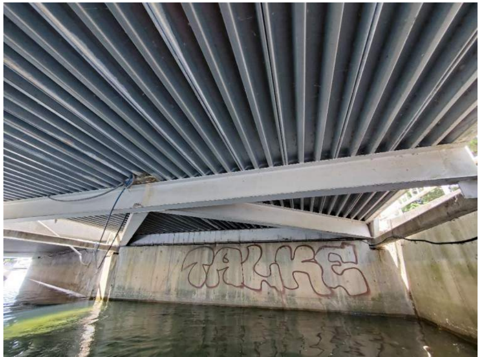
Figure 110: View of Eastern Phoebe nest on girder underneath Bridge 2 (B2). June 23, 2022.
