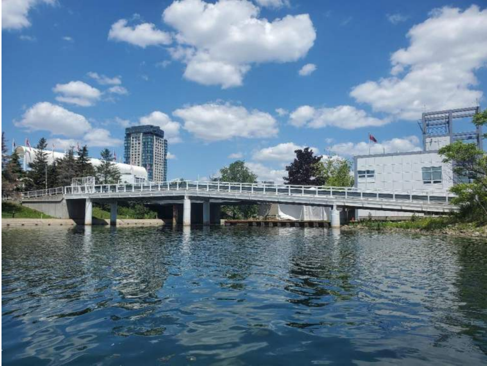
Figure 125: View, facing east, of Bridge 1A (B1A) and Bridge 1 (B1). June 23, 2022.
