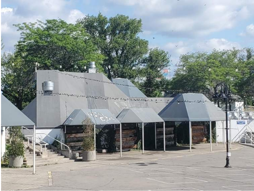
Figure 9: View, facing north, of Commons Food Building (B92547) on West Island, where Barn Swallows and American Robins nest under awnings. Hundreds of Cliff Swallows can be seen perched on strings of lights. July 12, 2022.
