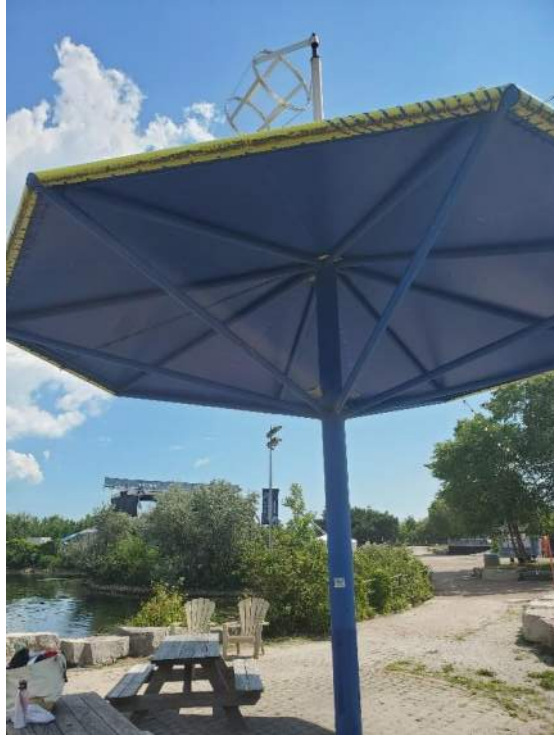
Figure 133: View, facing east, of patio and umbrella structure east of the Round Hut (B92563). August 24, 2022.
