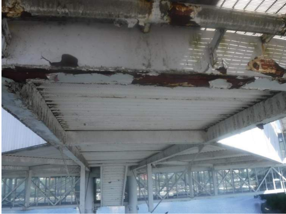
Figure 81: View of Cliff Swallow nests built on the underside of the Pavilion Pods (B92549 - 1-5). June 16, 2022.
