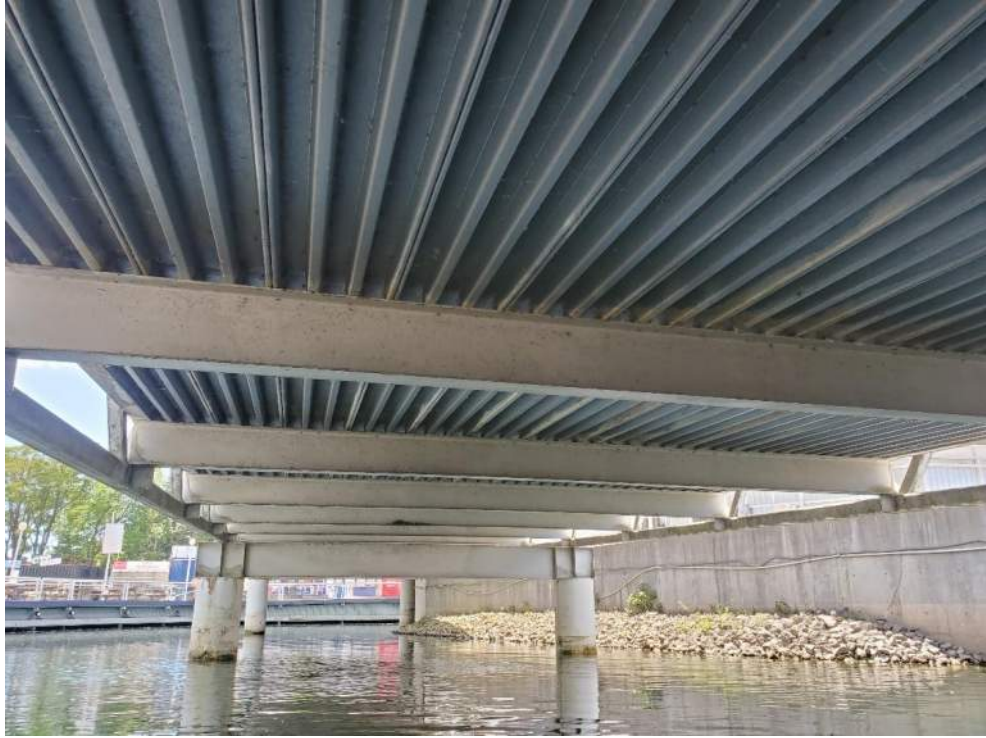
Figure 109: View, facing southwest, of the underside of Bridge 2 (B2). June 23, 2022.
