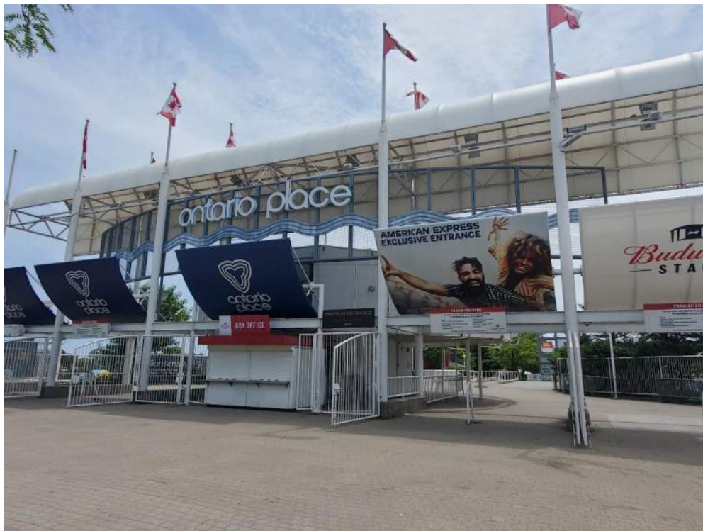
Figure 144: View, facing southeast, of the Central Entrance Structure (B92533). June 20, 2022.
