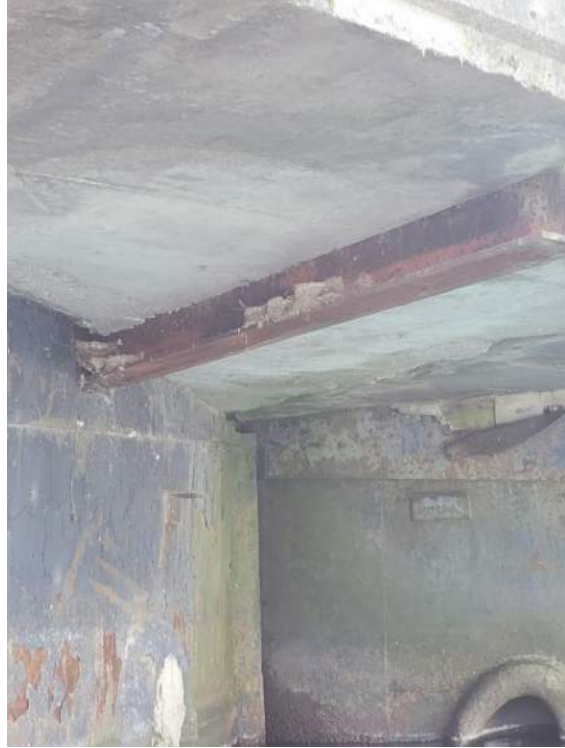
Figure 71: View of Barn Swallow nests on metal girder on Breakwater (BW). June 23, 2022.
