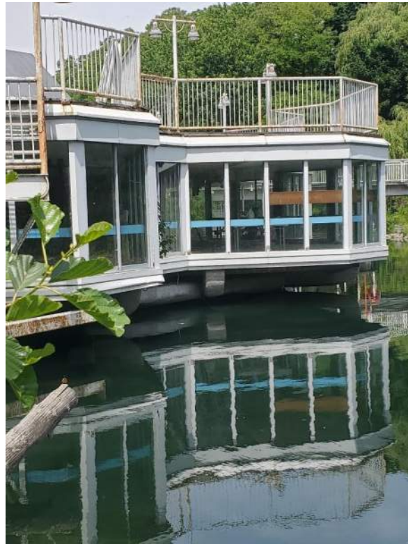
Figure 92: View, facing northwest, of the Marina North East Building (B92555) providing Barn Swallow nesting habitat where building extends over water, and directly on windows. June 20, 2022.
