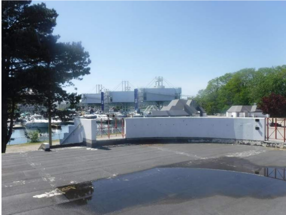
Figure 95: View, facing northwest of the sitting area on top of the Marina East Washroom Building (B92554).
