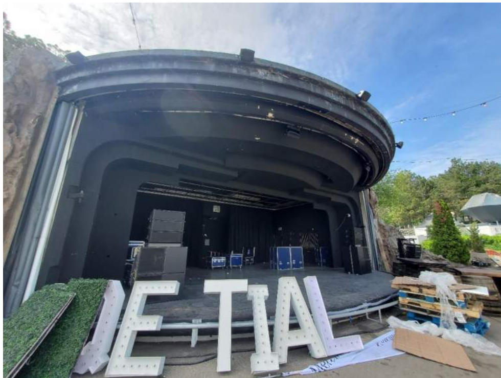
Figure 18: View, facing south, of the front of the Waterfall Stage (B92545). June 20, 2022.
