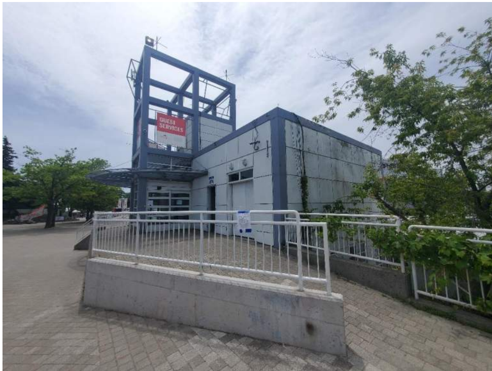
Figure 130: View, facing south, of the Centre Entrance Guest Services Building (B92567). June 20, 2022.
