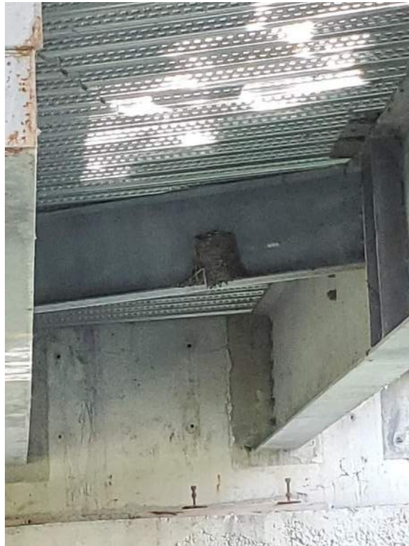
Figure 102: View of Barn Swallow nest on girder of Bridge 2 (B2A). June 23, 2022.
