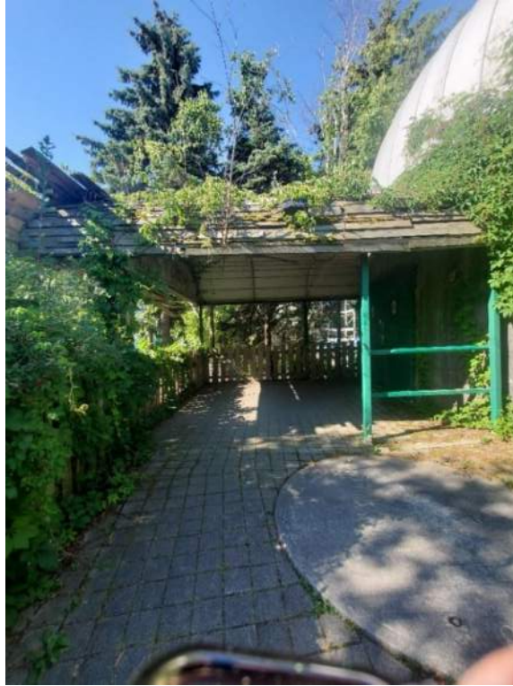
Figure 43: View, facing south, of covered entrance to the Interconnected Silos Complex at B92538-9. July 12, 2022.
