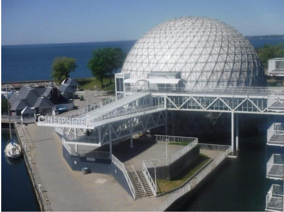
Figure 51: View of the Secondary Tower Ramp Element (SB7) leading to the Cinesphere (B92569) and Bridge 10 (B92572).
