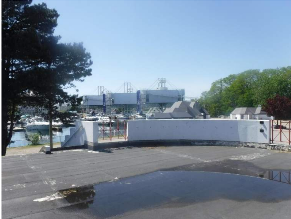
Figure 95: View, facing northwest of the sitting area on top of the Marina East Washroom Building (B92554).
