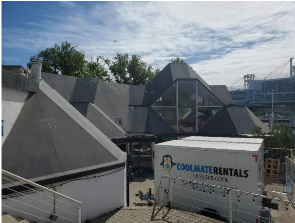
Figure 10: View, facing northeast, of Commons North East Building (B92581). June 20, 2022.
