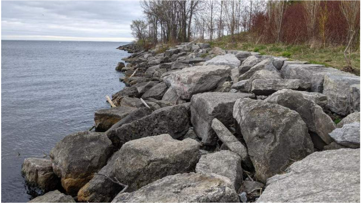
Figure 167: View of EIS-1 - Open Water Protected Sloped Shoreline habitat. May 5, 2021.
