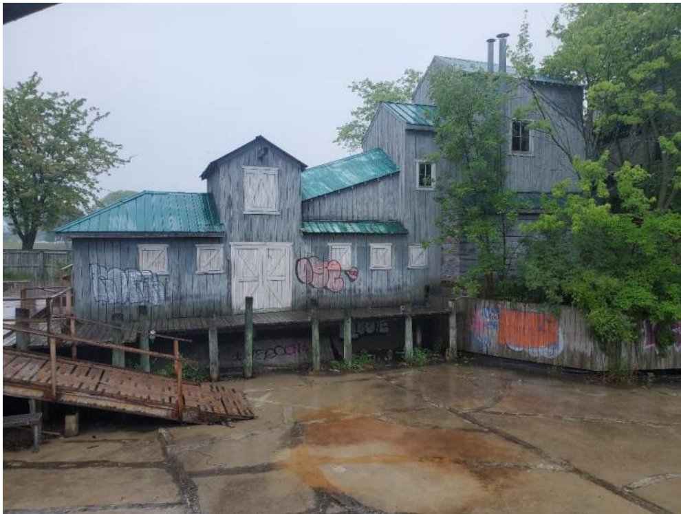
Figure 28: View, facing north, of the Ride Maintenance Building (B92540). July 5, 2022.
