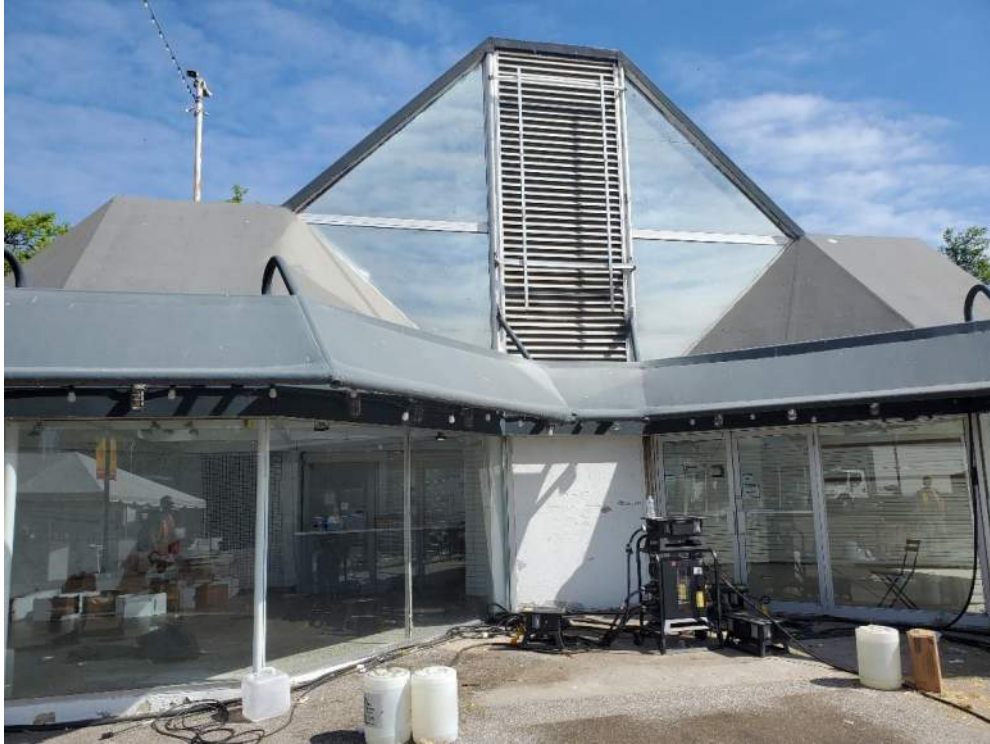
Figure 11: View, facing north, of Commons North Building (B92548). June 20, 2022.
