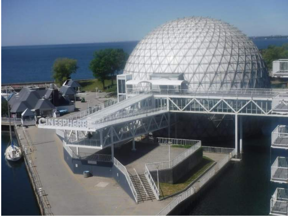
Figure 51: View of the Secondary Tower Ramp Element (SB7) leading to the Cinesphere (B92569) and Bridge 10 (B92572).
