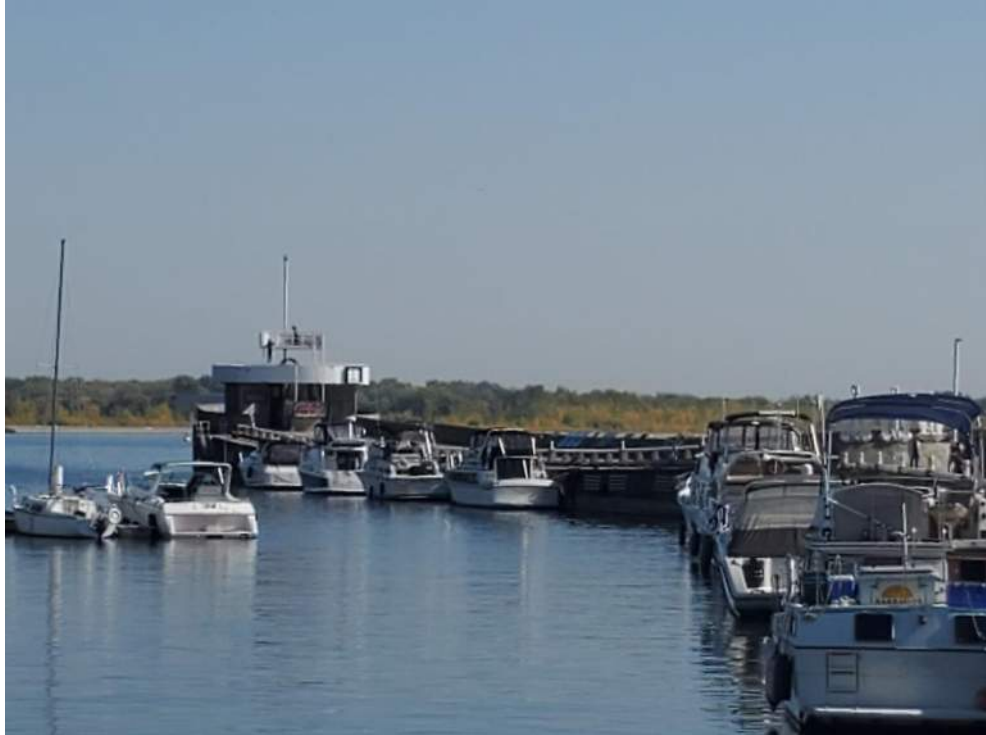
Figure 73: View, facing east, of the east end of the Breakwater (BW) with a viewing platform that provides a nesting area for Barn Swallows. October 11, 2022.
