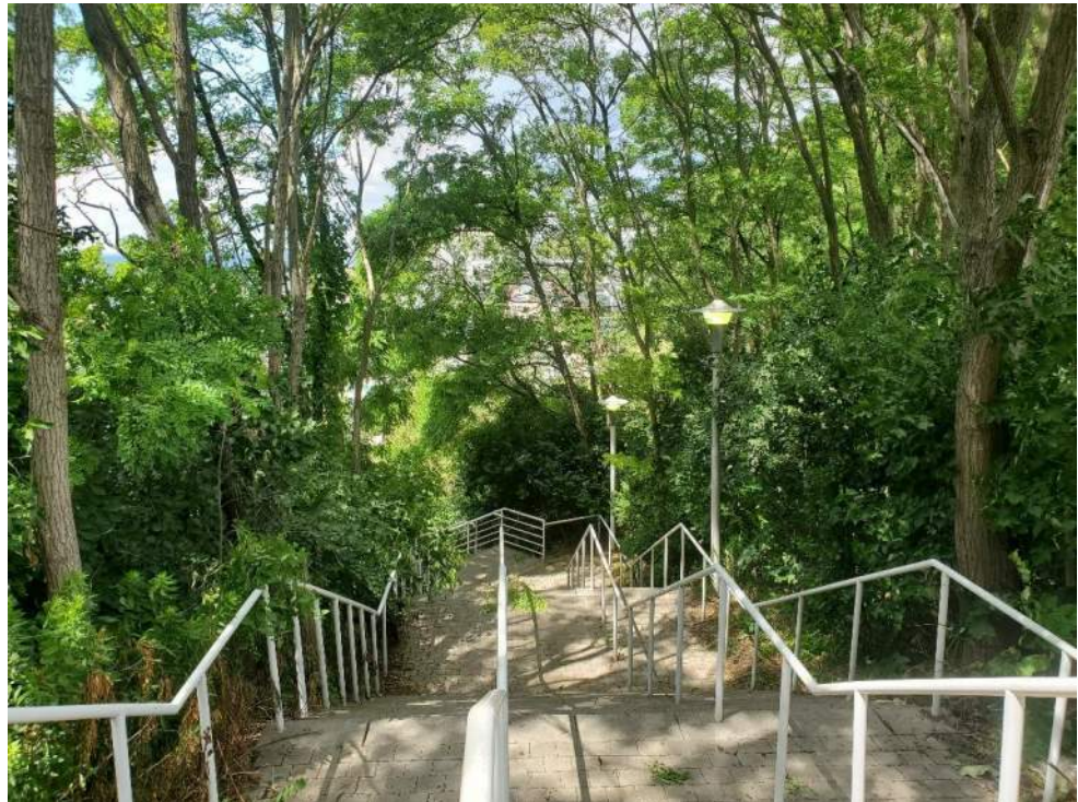
Figure 116: View, facing south, of the stairs from the Budweiser Stage lawn leading to Bridge 4 (B4). The stairs go through Vegetation Survey Area G. July 12, 2022.
