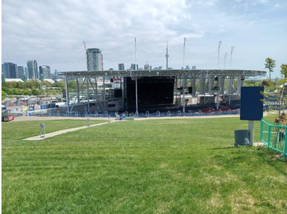
Figure 113: View, facing northeast, of the Budweiser Stage and lawn in Live Nation limits. May 25, 2022.
