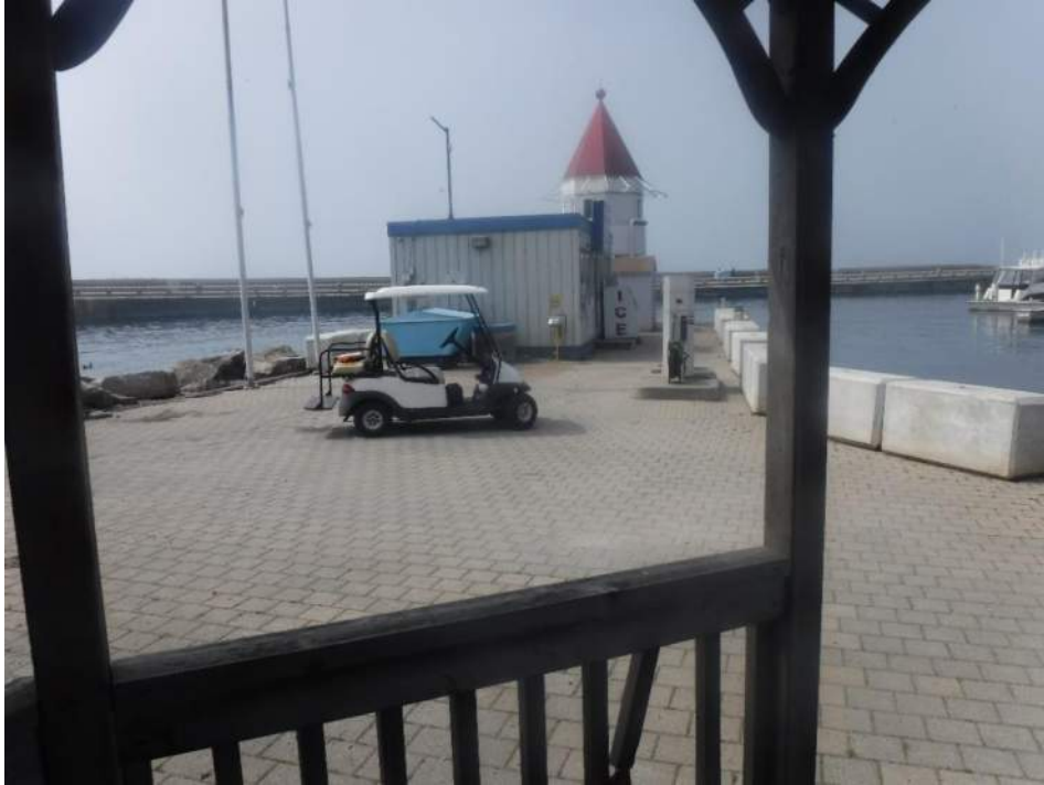
Figure 97: View, facing south, of the Marina East Tuck Shop (B92553) and Marina East Lighthouse (B92552).
