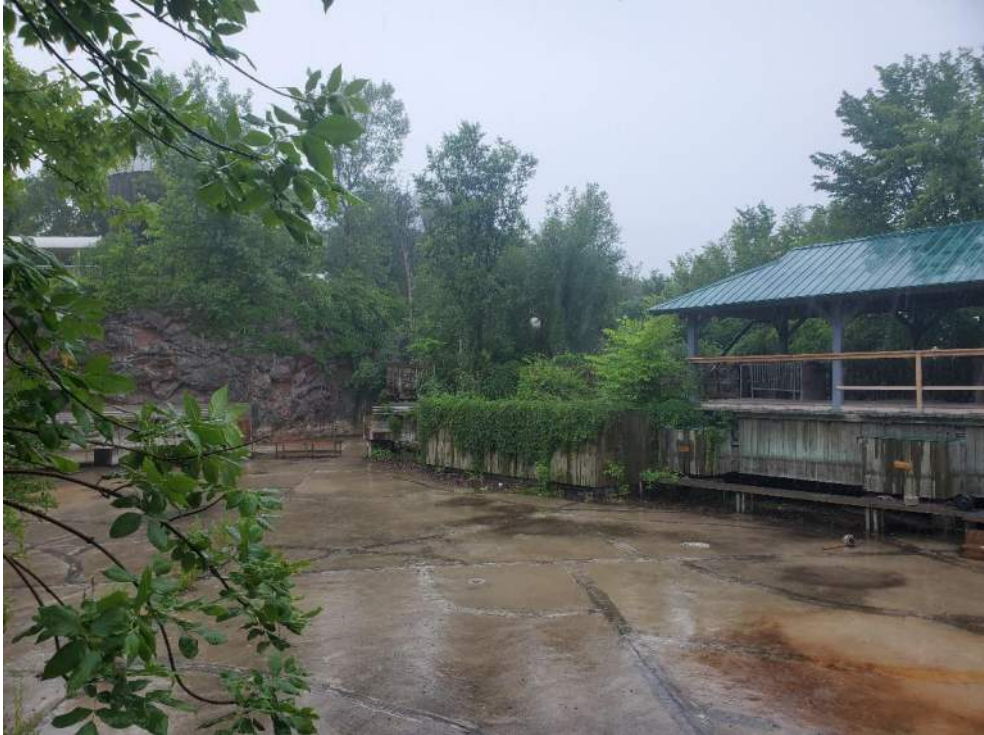
Figure 31: View, facing south, of the Ride Maintenance Building (B92540) area, showing Vegetation Survey Area J in the background. July 5, 2022.
