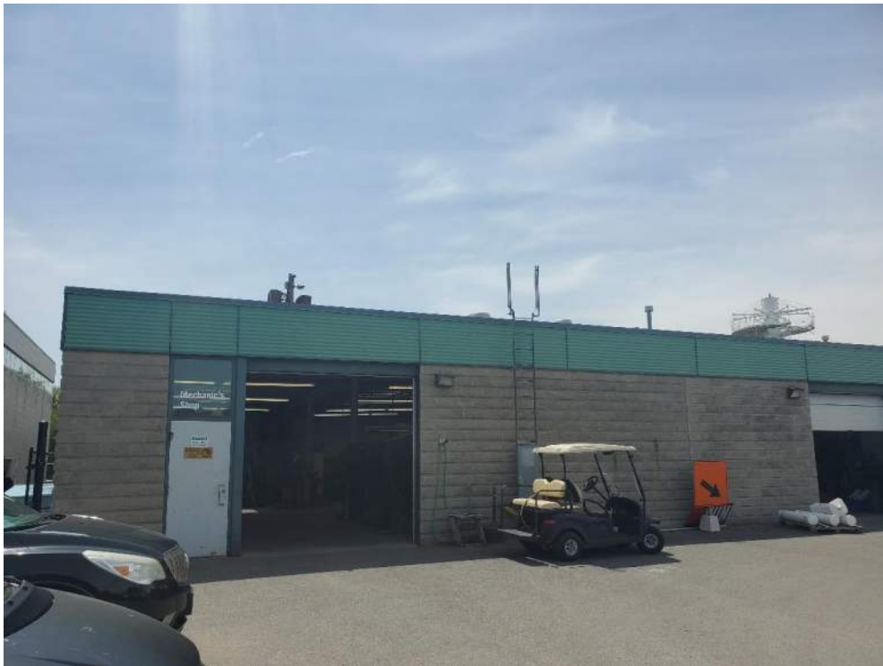
Figure 140: View, facing south, of the Maintenance Building (B92579). June 20, 2022
