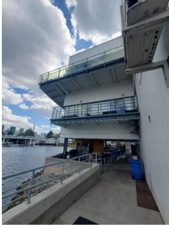
Figure 119: View, facing east, of Live Nation decks and lounges on the north side of the Budweiser Stage. July 12, 2022.
