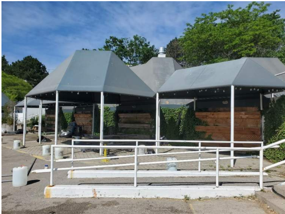
Figure 12: View, facing northwest, of Commons Food Building (B92547) where Barn Swallows and American Robins nest under awnings. June 20, 2022.
