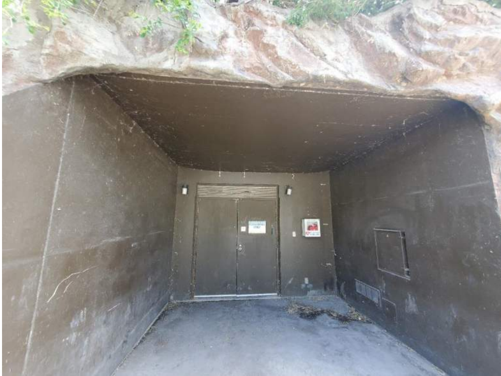
Figure 19: View, facing east, of the side of Waterfall Stage Building (B92545). June 20, 2022.
