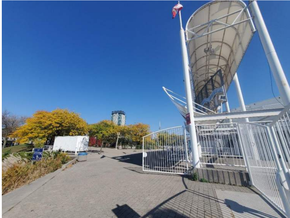
Figure 145: View, facing northeast, of the Central Entrance Structure (B92533) and Bat Acoustic Monitoring Area #9. October 11, 2022.
