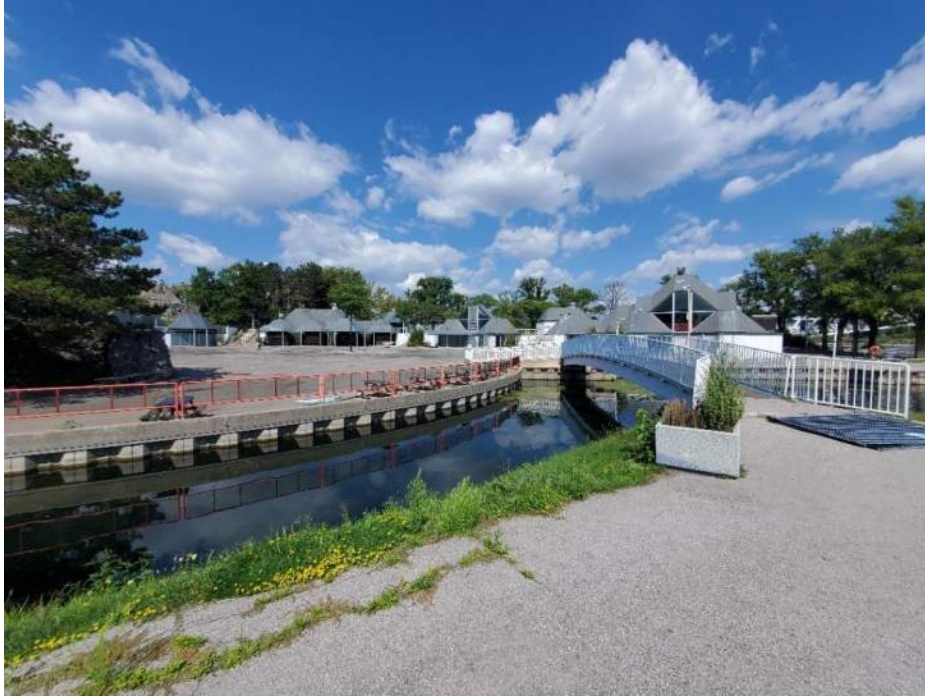
Figure 25: View, facing northwest, of the West Island Commons buildings and Bridge 13 (B13). June 20, 2022.
