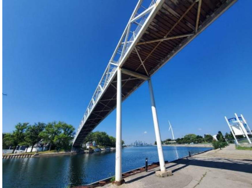
Figure 5: View, facing west, of Bridge 6 (B6) and Waterfowl/Shorebird Survey Area #6. May 20, 2022.
