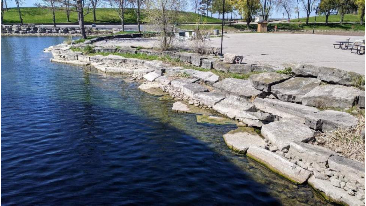
Figure 171: View of MB-3 – Marina Basin Protected Sloped Shoreline habitat. May 12, 2021.
