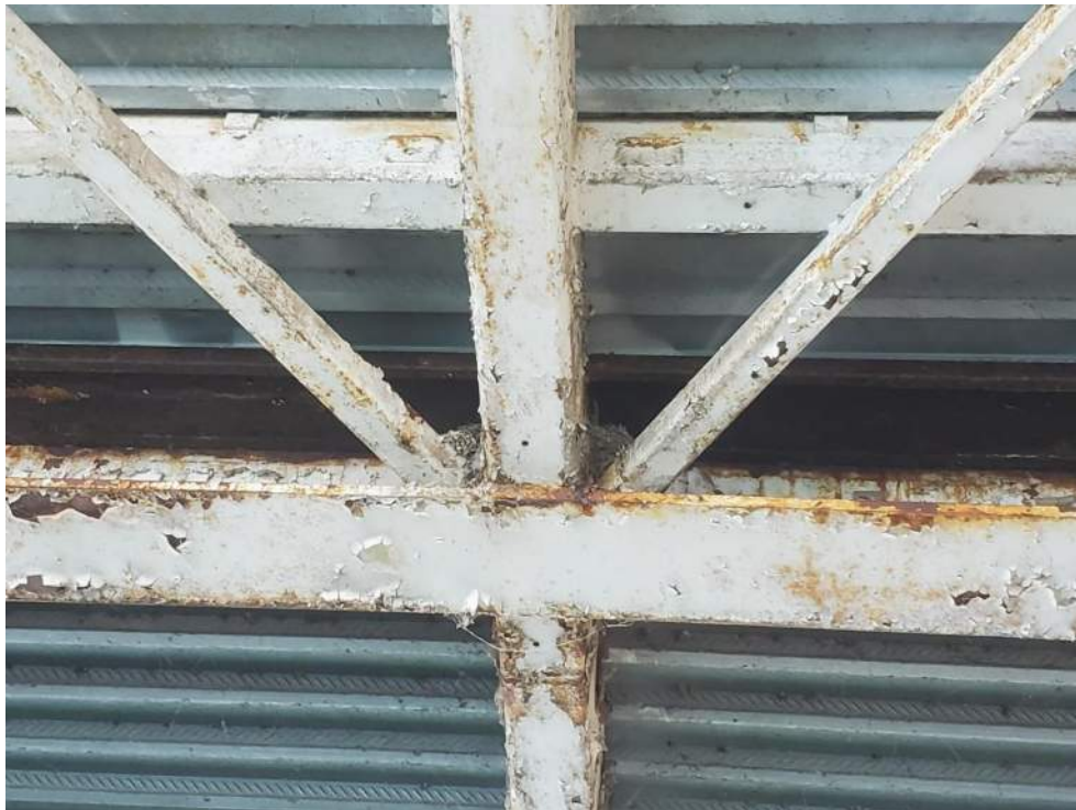
Figure 128: View of Barn Swallow nests on girders under Bridge 1 (B1). June 23, 2022.
