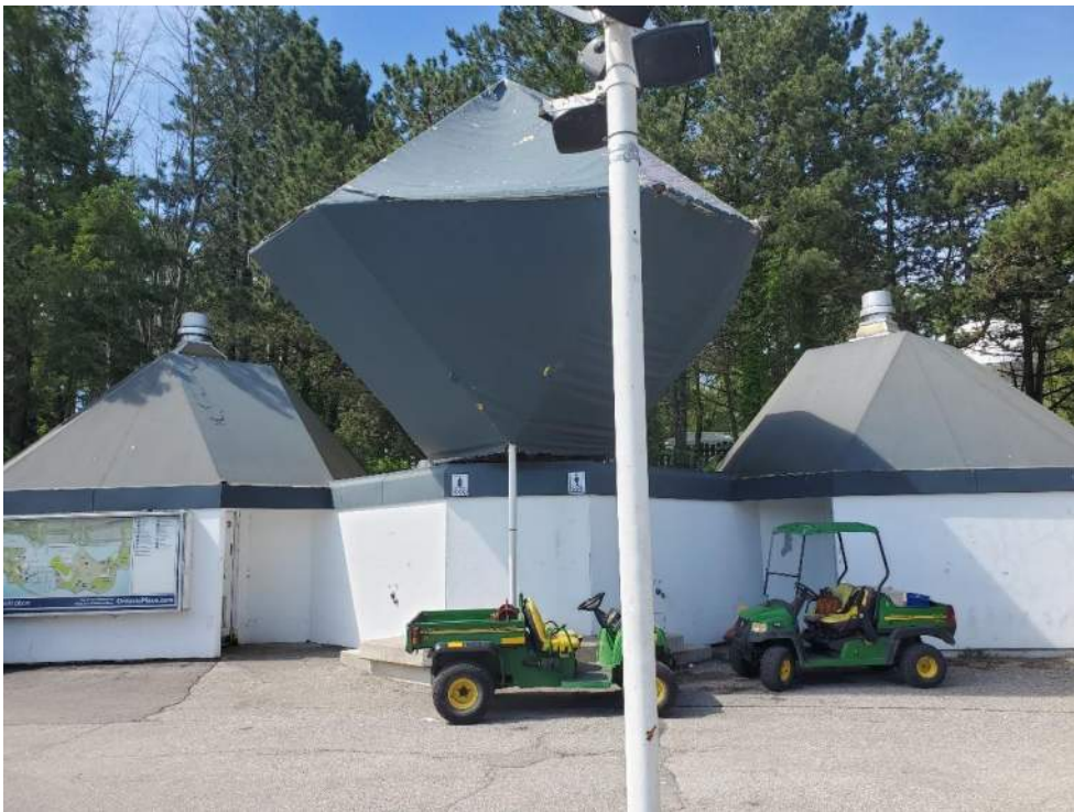
Figure 24: View, facing west, of the Commons South Washrooms (B92541). A portion of Landbird/Breeding Bird Survey Transect #6 is also visible in the background. June 20, 2022.
