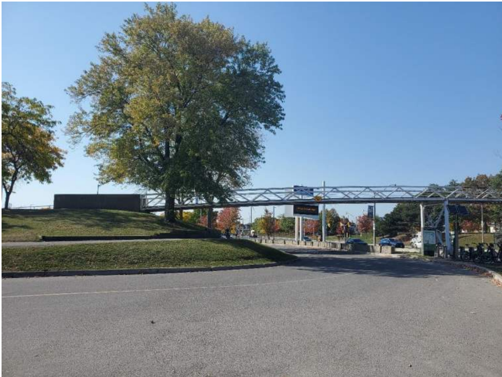
Figure 148: View, facing west, of Bridge 8 (B8). October 11, 2022.
