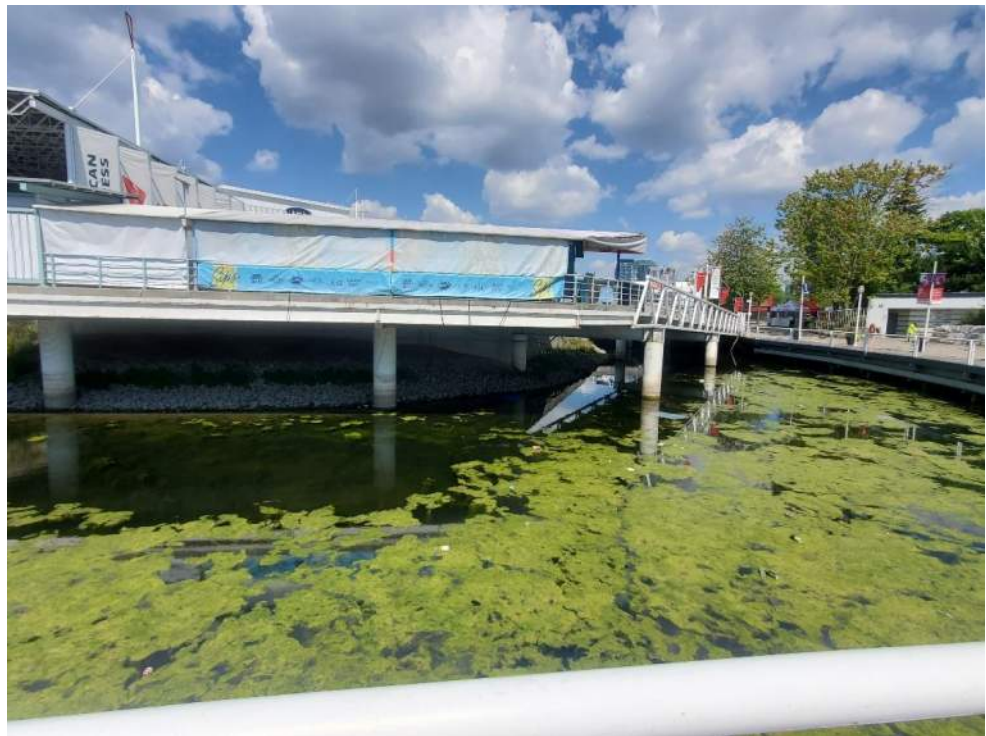
Figure 106: View, facing north, of Live Nation deck over water providing Barn Swallow nesting habitat southwest of Bridge 2 (B2). Algae bloom in channel also visible August 24, 2022.
