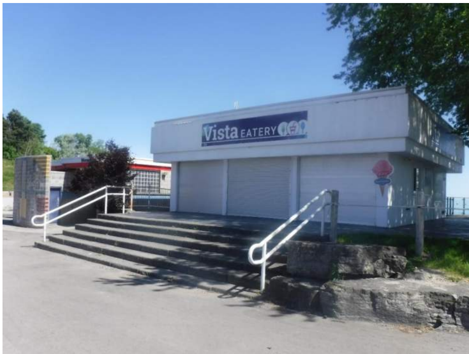
Figure 98: View of the East Island South Building (B92566) and the East Island South Washroom (B92565). June 5, 2022.
