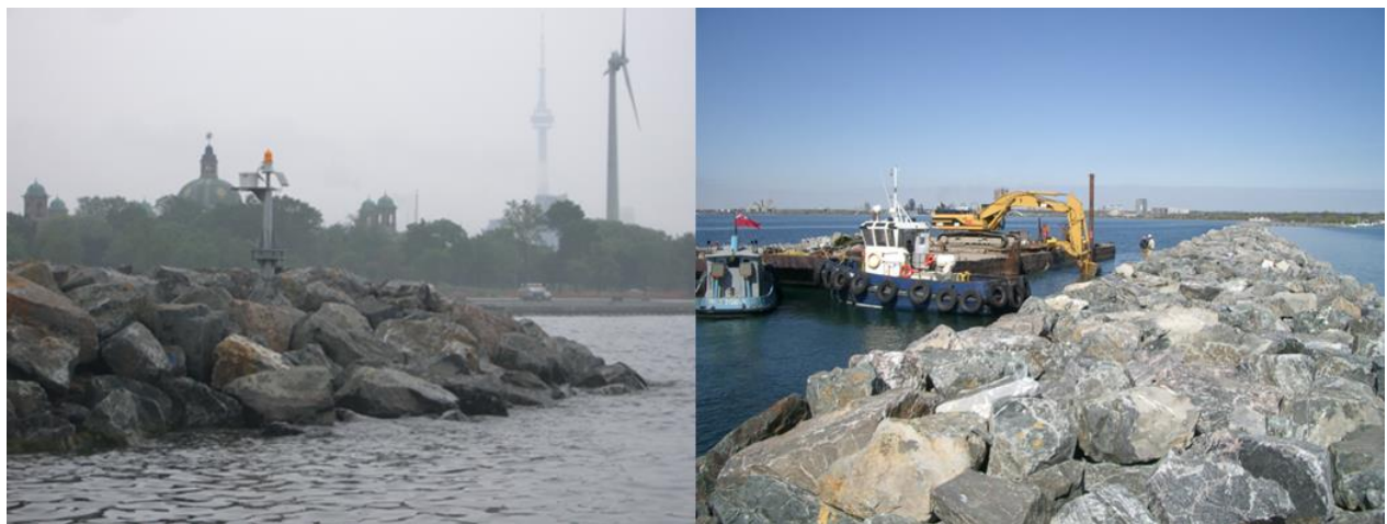
Figure 14: Armour protection at Western Beaches breakwater (Baird)
