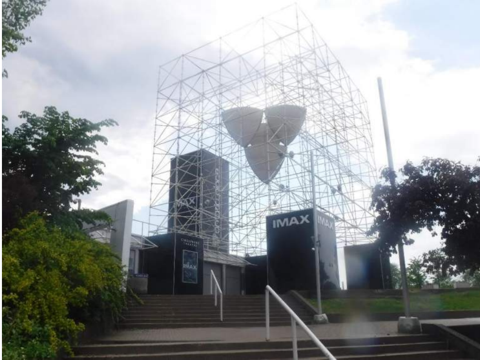
Figure 1: View, facing southwest, of the West Entrance Building (B92580). June 5, 2020.
