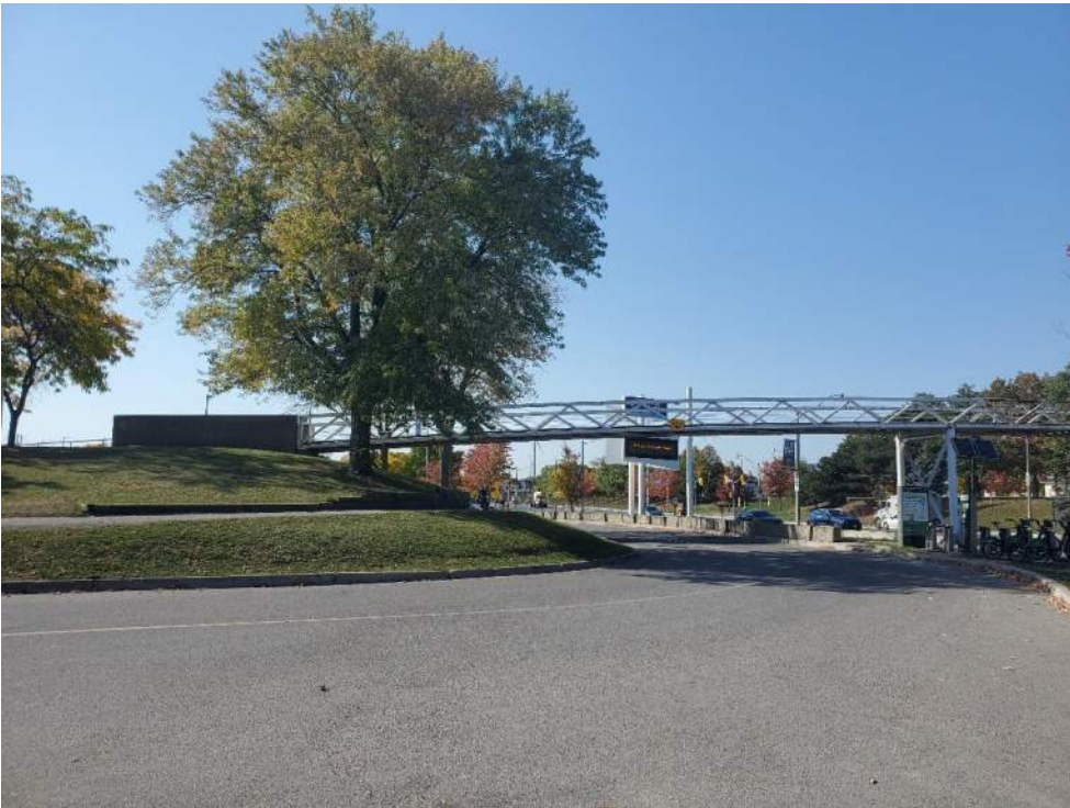
Figure 148: View, facing west, of Bridge 8 (B8). October 11, 2022.
