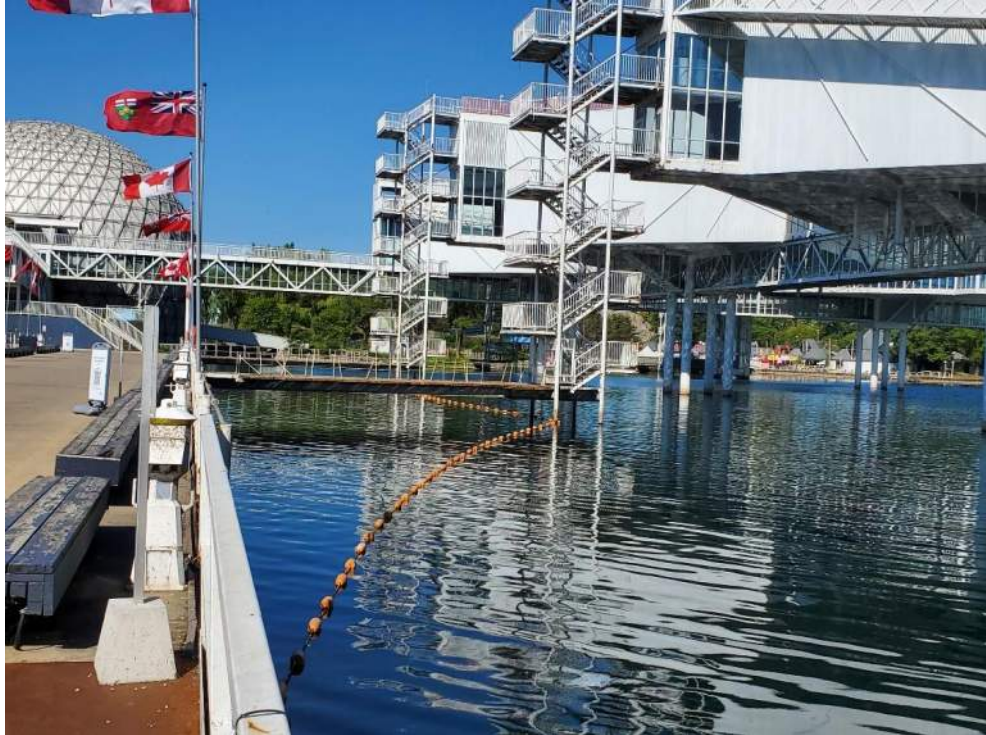
Figure 85: View, facing west along Bridge 5 (B92575), of Secondary Bridge 3 (SB3) and Secondary Bridge 4 (SB4), each providing nesting habitat for Barn Swallows. August 24, 2022.
