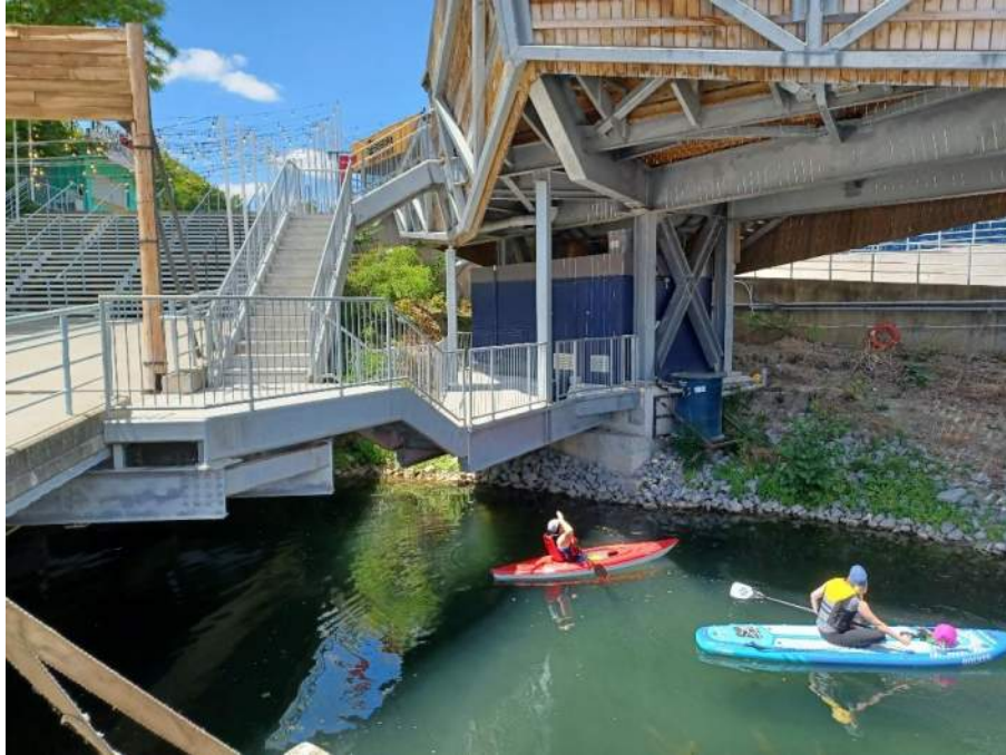
Figure 101: View, facing west, of Bridge 2A (B2A) providing Barn Swallow habitat. June 23, 2022.
