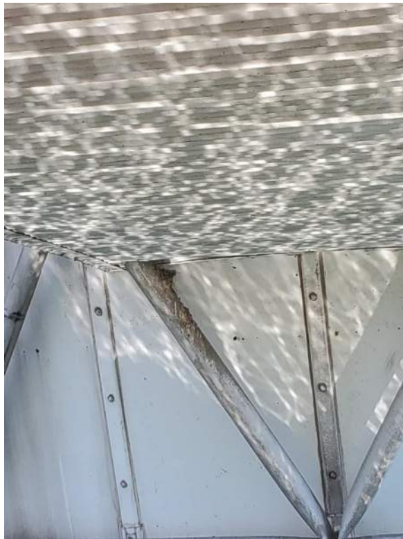
Figure 52: View of Barn Swallow nest under Secondary Ramp Element 6 (SB6). June 23, 2022.
