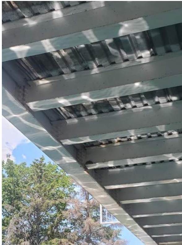
Figure 126: View of a Barn Swallow nest on a girder on Bridge 1A (B1A). June 23, 2022.
