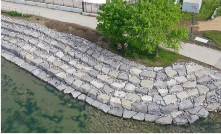
Figure 17: Example of terraced armour stone at Sunnyside (photo courtesy TRCA)
