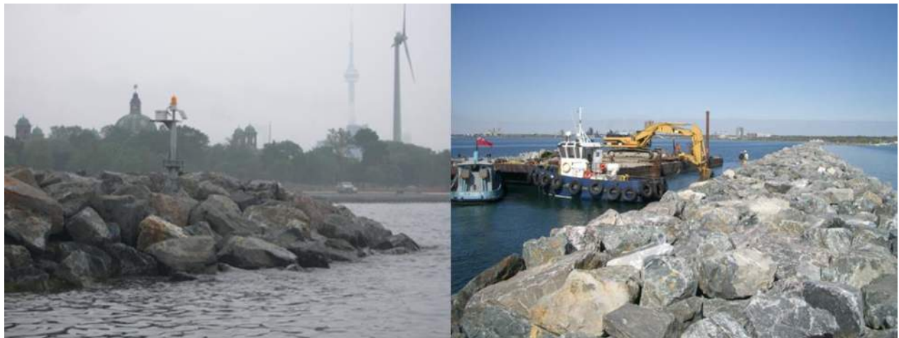
Figure 14: Armour protection at Western Beaches breakwater (Baird)
