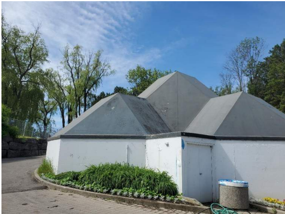
Figure 20: View, facing west, of the Electrical Sub Station Building (B92544). June 20, 2022.
