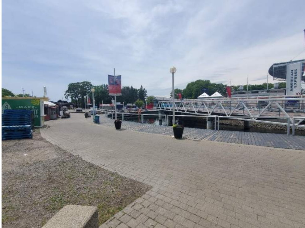
Figure 105: View, facing southwest, of Bridge 2 (B2) and surrounding walkways. June 20, 2022.
