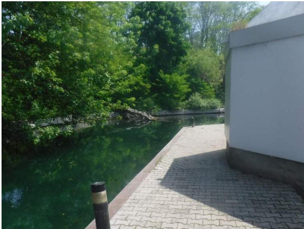
Figure 88: View, facing east, of Landbird/Breeding Bird Survey Transect #9 and Marina North Washroom Building (B92556). June 5, 2020.
