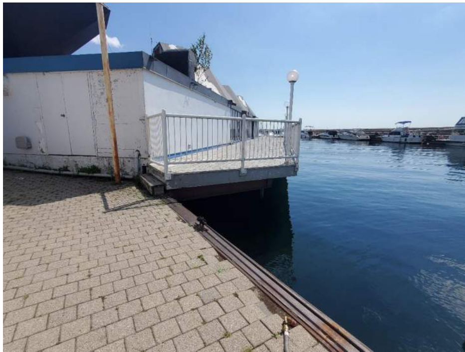
Figure 66: View, facing east, of West Marina Village Building (B92550) deck that provides Barn Swallow nesting habitat underneath, and of Waterfowl/Shorebird Survey Area #3. June 23, 2022.
