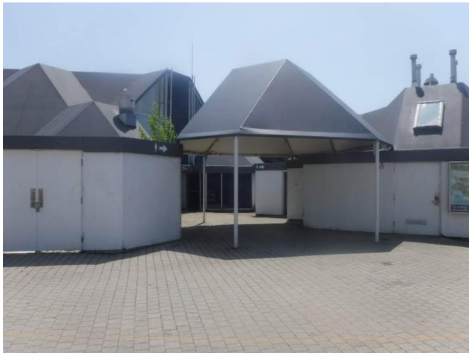
Figure 58: View, facing south, of the Marina West Washrooms (B92551) and the West Marina Village Building (B92550). June 5, 2020.
