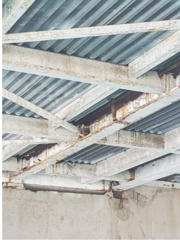
Figure 129: View of Barn Swallow nest on girders under Bridge 1 (B1). June 23, 2022.
