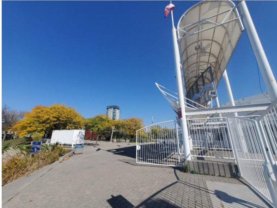
Figure 145: View, facing northeast, of the Central Entrance Structure (B92533) and Bat Acoustic Monitoring Area #9. October 11, 2022.
