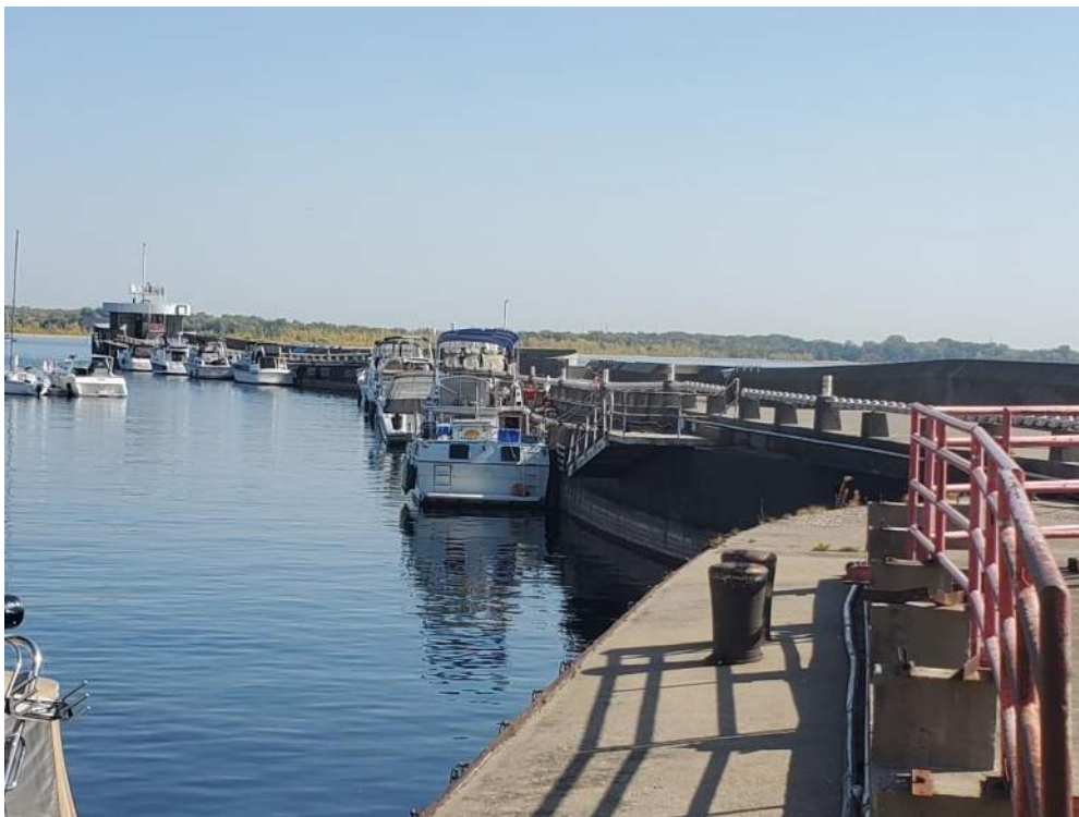
Figure 68: View, facing east, of the Breakwater (BW). October 11, 2022.
