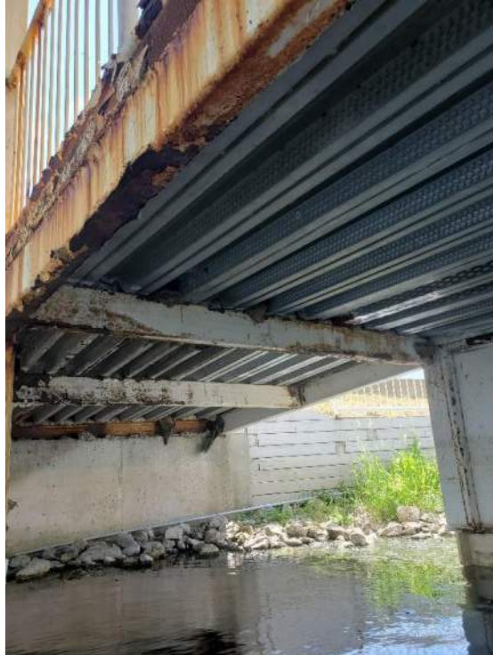
Figure 53: View, facing southeast, of prevalent Barn Swallow nesting under Secondary Tower Ramp Element 7 (SB7) at Cinesphere (B92569). June 23, 2022.
