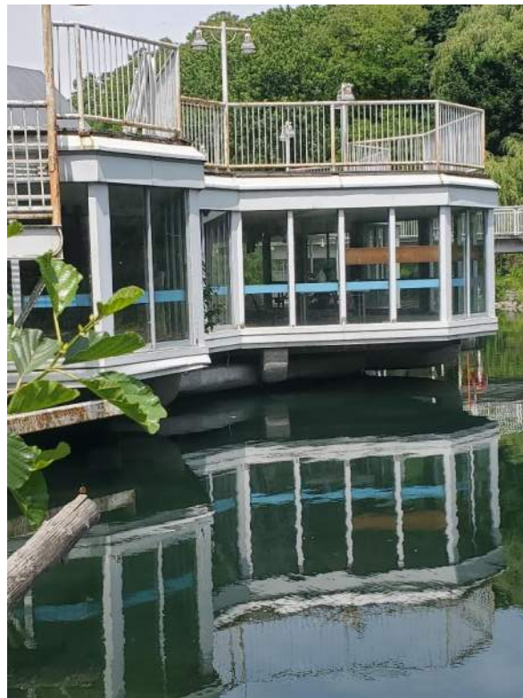
Figure 92: View, facing northwest, of the Marina North East Building (B92555) providing Barn Swallow nesting habitat where building extends over water, and directly on windows. June 20, 2022.
