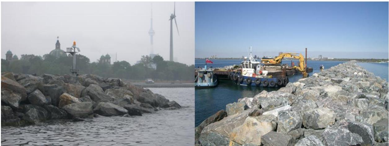
Figure 14: Armour protection at Western Beaches breakwater (Baird)
