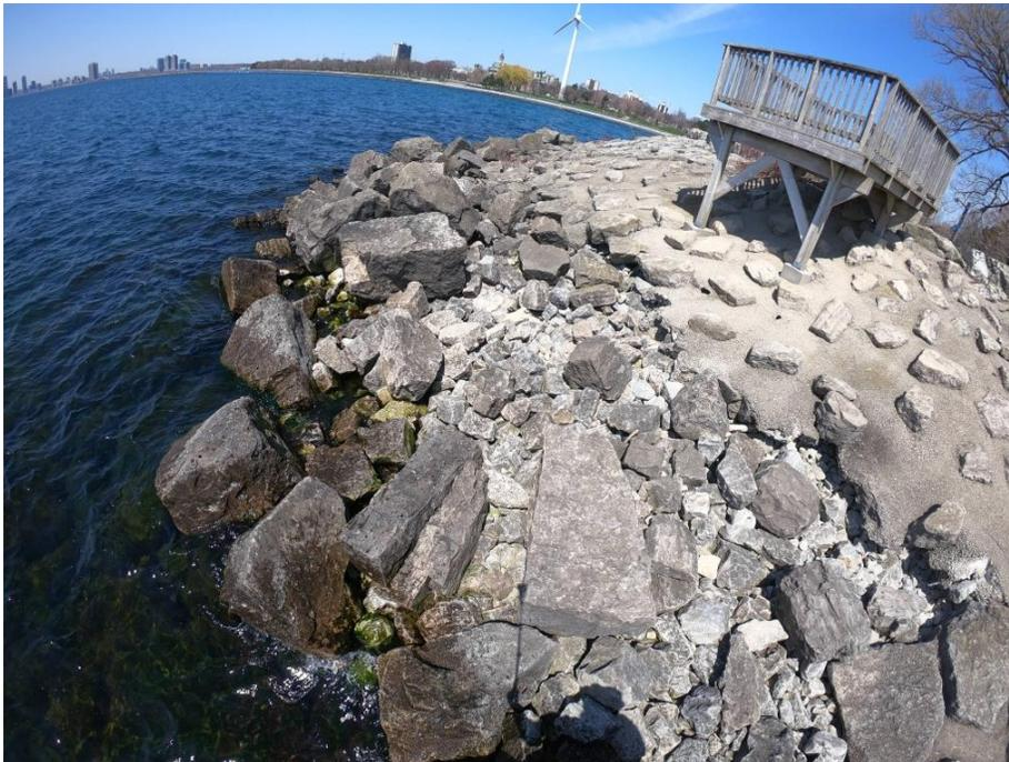
**Figure 9: Damaged armour protection at west headland (Baird 2022-04-29)**
