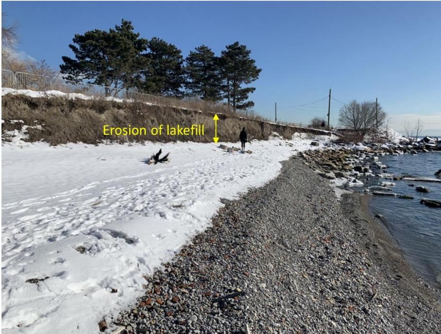
Figure 10: Significant erosion of lakefill at south shore (Baird 2021-01-30)
