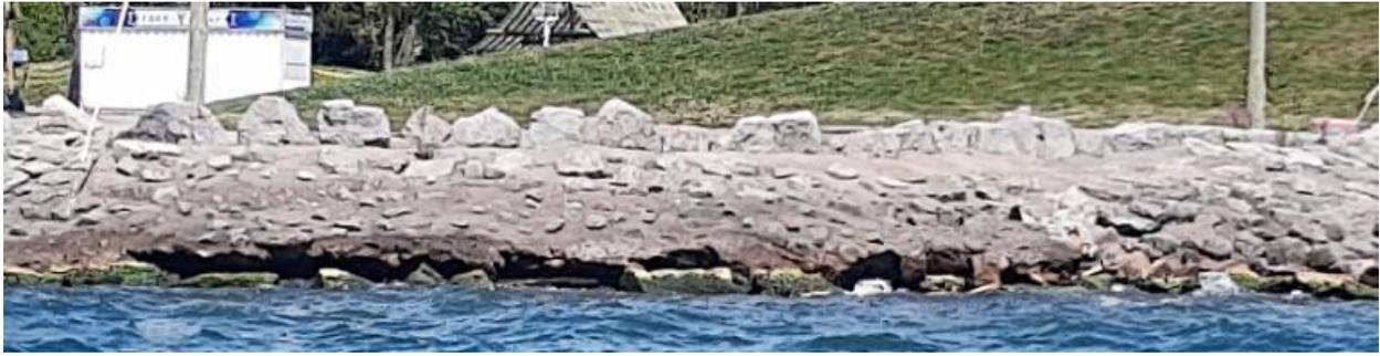
**Figure 12: Deterioration of grouted stone revetment at east headland (from Jacobs, 2020)**
