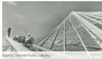
1970 ZEIDLER PODS NEAR COMPLETION
